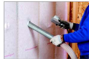
Finishing the system with PINK FIBERGLAS™ Blown-In Insulation of the EnergyComplete™ system delivers exceptional energy efficiency and acoustical performance.
