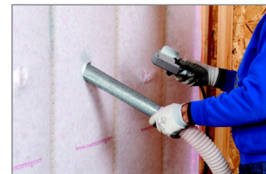
The EnergyComplete™ system delivers exceptional energy efficiency and acoustical performance, when finished with PINK FIBERGLAS™ blown-in Insulation shown here.
