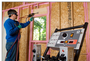
The PINK foam-based air sealing component of the EnergyComplete™ system helps reduce air infiltration by up to 70 percent.
